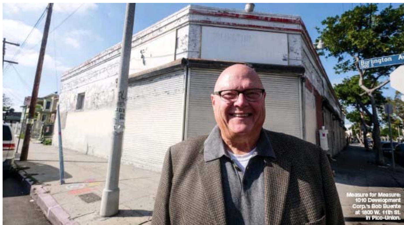
Measure for Measure: 1010 Development Corp.'s Bob Buente at 1800 W. 11th St. in Pico-Union.
